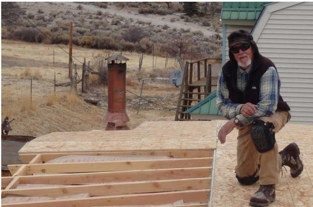
In early November the south trailer began to get a much-needed new roof. The original roof was nearly 50 years old, and in addition to leaking in several places, it lacked insulation. The new roof, tar-papered and not yet shingled, has withstood the wind and snow. The additional insulation has made a huge difference in terms of heating bills and inside comfort. When the weather clears, the shingles will be stapled on to finish up the project.
